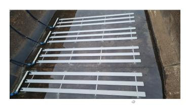
A special feature of this plant is the shallow water depth of 2.0 m in carousel 1 and 2.7 m in carousel 2. With a measured oxygen utilization (SSOTR) of more than 35 g/Nm³mid the AEROSTRIP® modules quickly pay for themselves even under these conditions.
