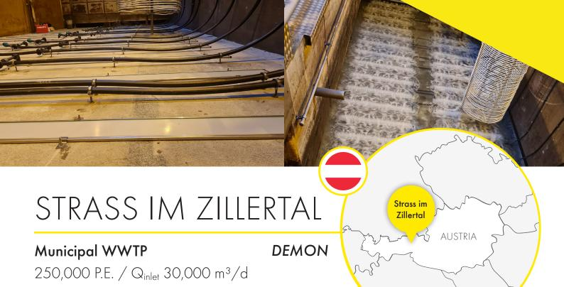
The Strass wastewater treatment plant in the Zillertal valley treats wastewater from the tourist-oriented valleys of Achental, Inntal and Zillertal (AIZ) and has been energy self-sufficient since 2005. The same year the DEMON method for treating process water was implemented for the first time, resulting in more energy production then the plant consumes.
